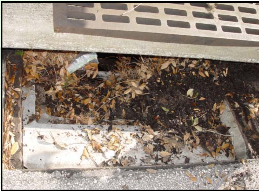
View of inlet filter immediately after grate was removed.
