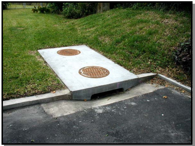
Finished Project along Weber St., Orlando, FL
