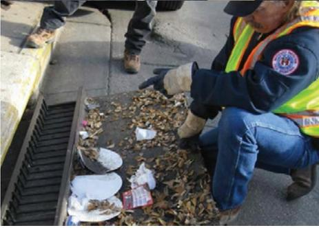
The outdated inlet filter traps that were previously installed in 6th Street are inefficient, cumbersome and can often be difficult and dangerous to service.
