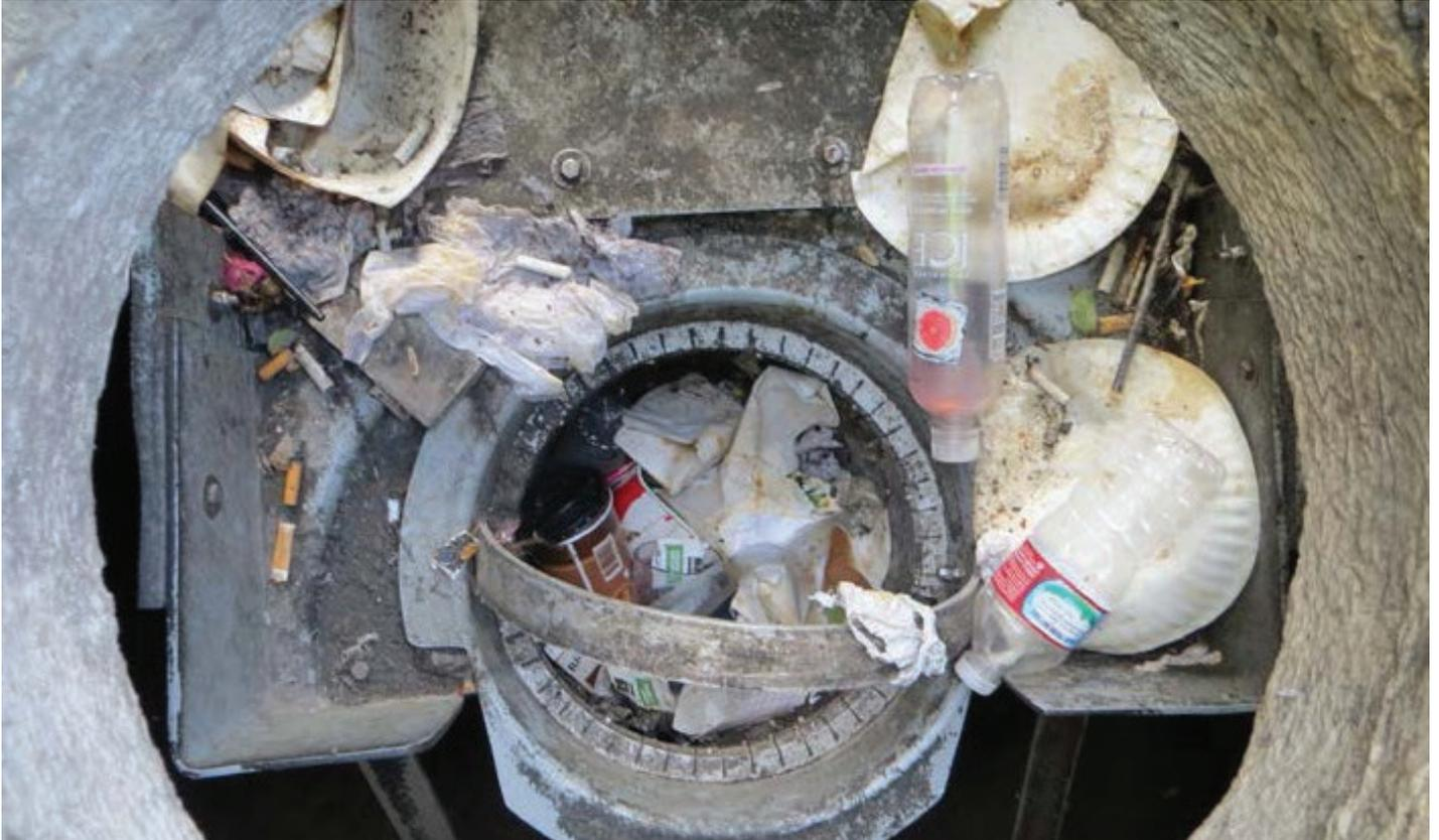
One of many High Capacity Curb Inlet Basket™ inlet filters full of captured trash and sediment within a 6th Street catch basin. The Suntree High Capacity Curb Inlet Basket is able to be custom constructed to adapt to any type or size manhole access and is far more efficient at capturing and containing gross solid pollutants compared to the older inlet filter trap devices.
