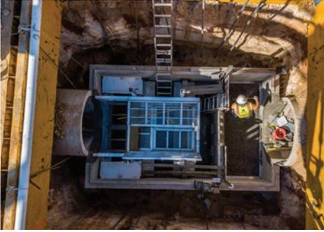
Installation personnel work on completing the upflow filtration chamber by installing the Bold & Gold biosorption media bed.
