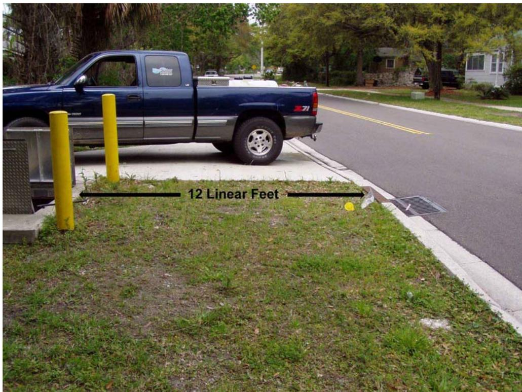
Deliver the sand through the catch basin located at the curb using a 1/2 inch PVC tube. Position the PVC tube at the leading edge of the 24inch squat pipe where it leaves the catch basin to deliver the sand directly into the pipe and not the bottom of the catch basin.
