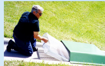
1 Remove Filter Insert
