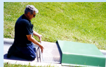
3 Replace Filter Insert
